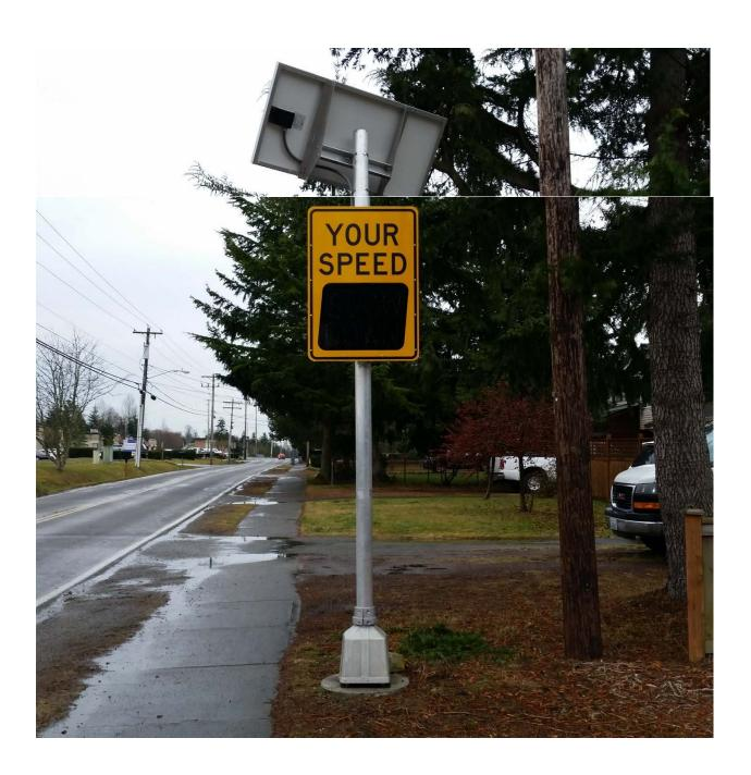
This sign is a edited representation of the signs Clyde Hill is installing. The posts are forrest green. The sign faces are white with black lettering. The bottom of the sign will be 7 feet above the adjacent street or sidewalk. The sign is three feet tall and the solar panel is 2 feet by 4 feet.
