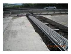
prestressed concrete structure has a length of 931 m. During the course of renovation works in 2009, the expansion joints at each end of its deck were renewed.
